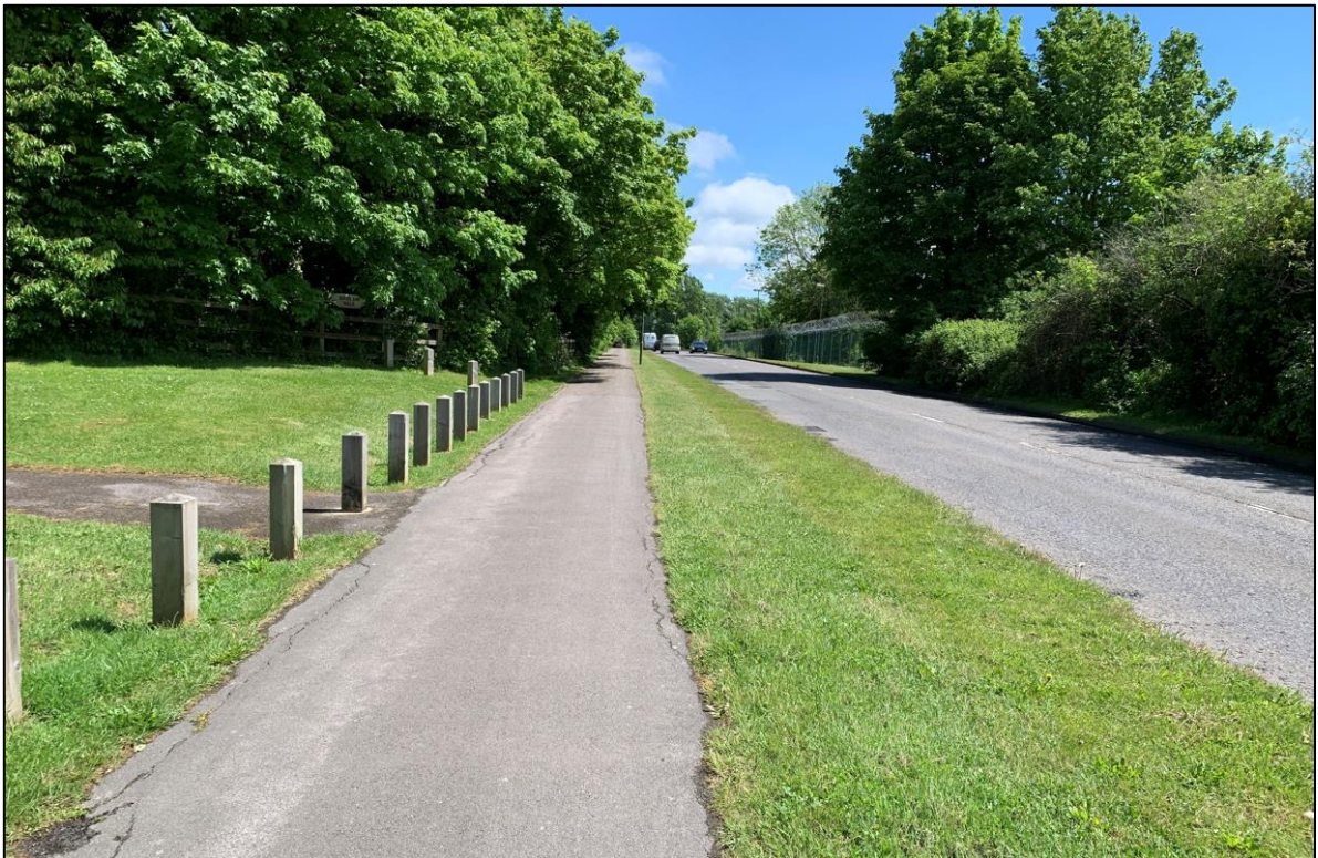
Image 1: Existing Footway Along Longfield Avenue
