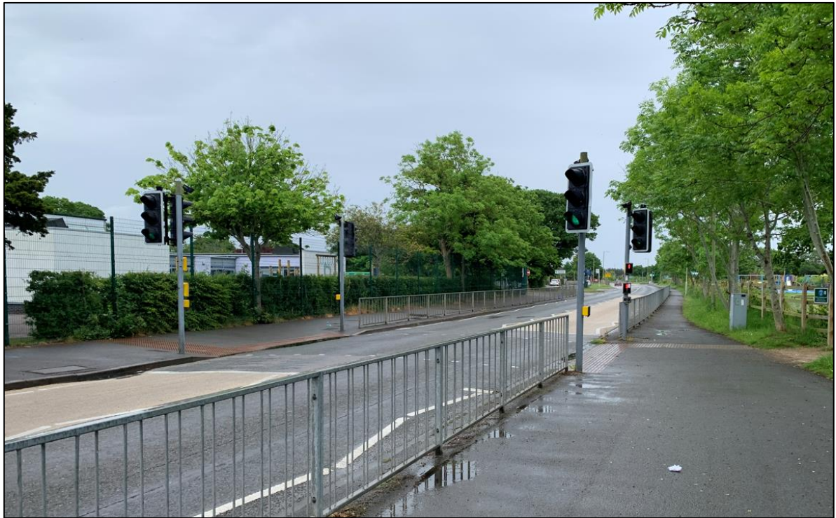
Image 4: Signal Controlled Crossing Across Gosport Road
