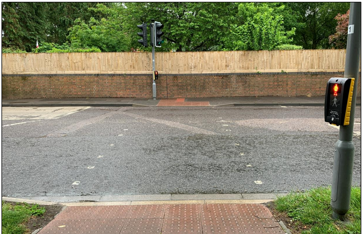
Image 5: Existing Signal Controlled Pedestrian Crossing Across Stubbington Lane
